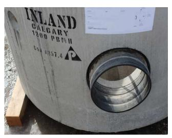
A smooth cored hole with a booted gasket connection is a water-tight design for flexible pipe.
