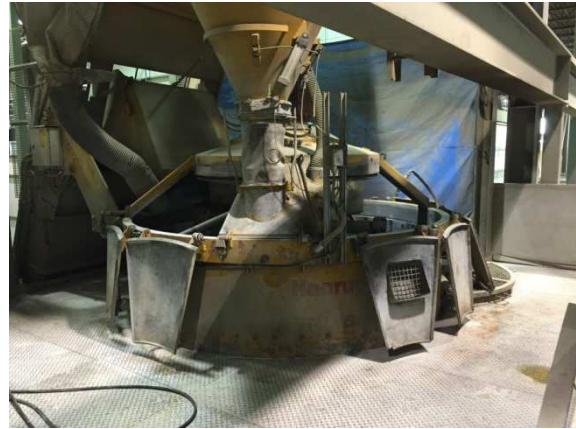
Figure 2: A concrete mixer at Inland's Spyhill Plant in Calgary
